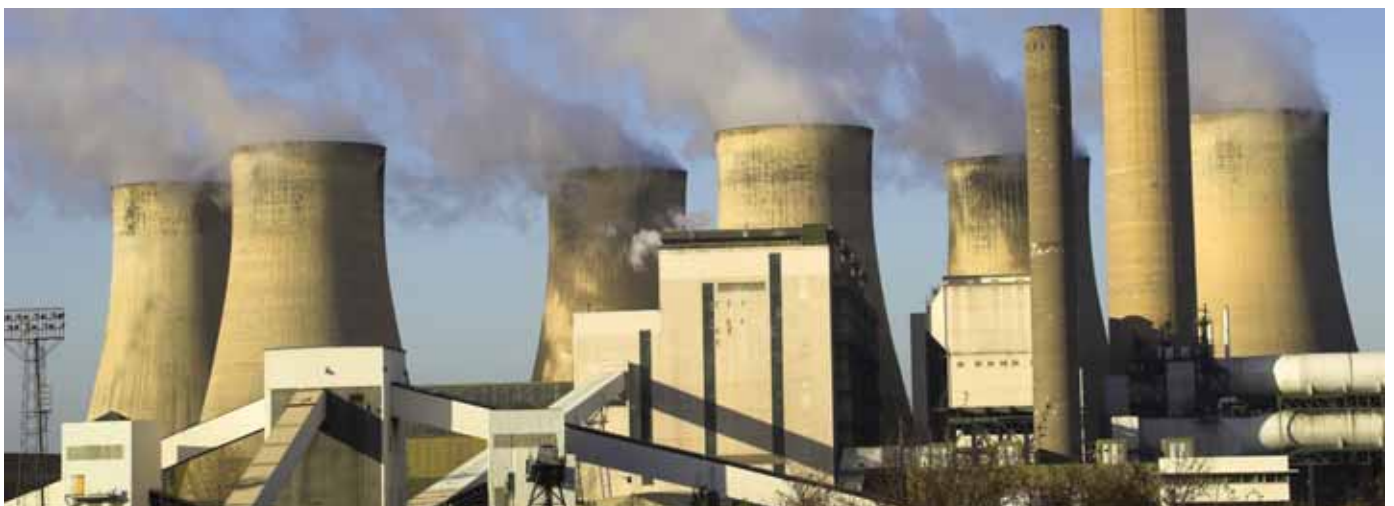
Coal Fired Power Station
